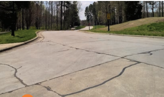
1 Davie Intersection before
