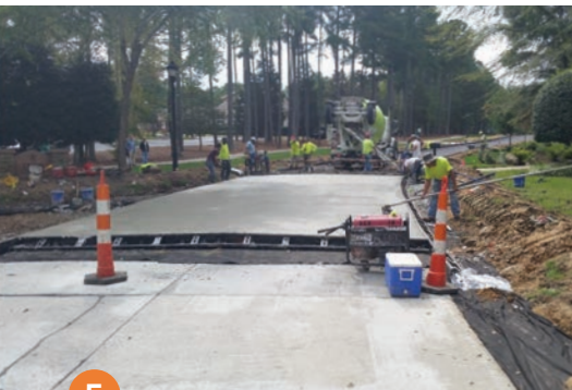
5 7-inch concrete overlay - Phase 2
