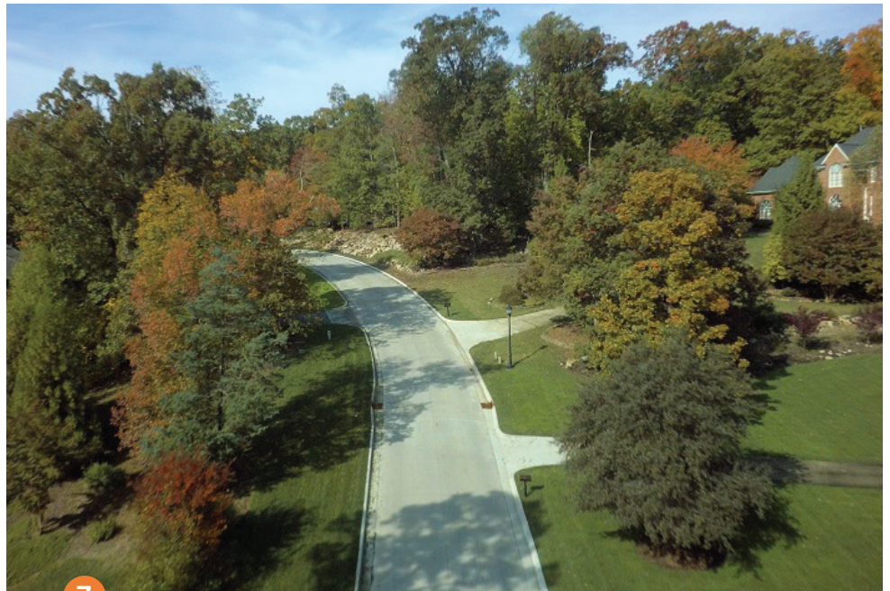
7 Completed concrete overlay
